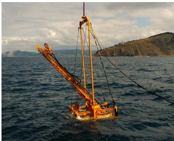
Fig 2. Remotely operated submarine drilling rig used for rotary boreholes
