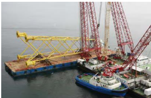
Fig. 1. Jacket structure on a barge.
