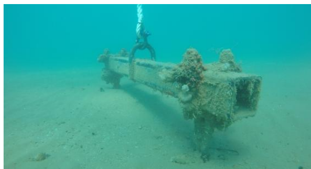
Fig. 2. Anchorage system for sandy substrate.
